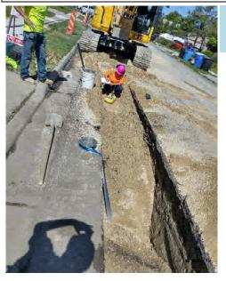
Taking density tests on the new backfill over the pipeline
