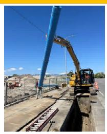
Installing new 12-inch pipeline
