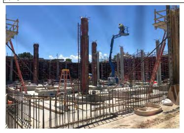
Final corner of the reservoir walls, columns, and floor to be finished
