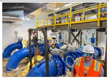
Modification of the discharge piping to eliminate air binding
