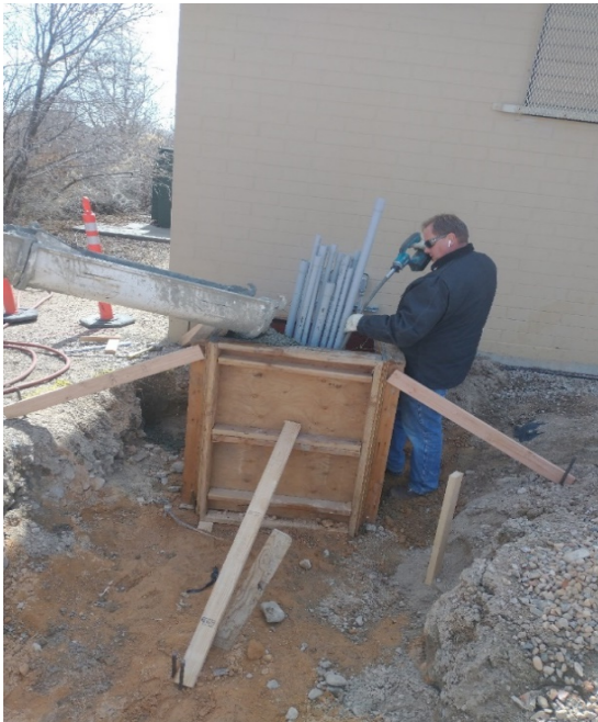
Pouring concrete for new RTU pedestal
