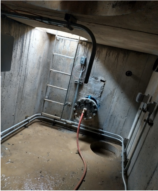
Old piping removed and awaiting new valves, meter, and pipeline
