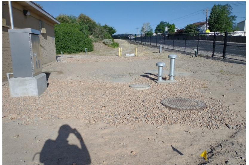
Completed job site with RTU cabinet, vents, and vault
