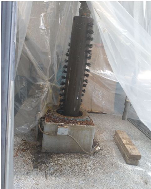
Brushing the well shaft
