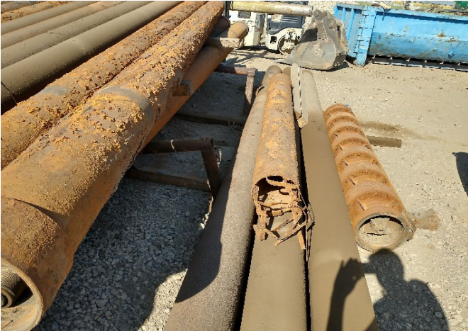
Condition of removed pump and column
