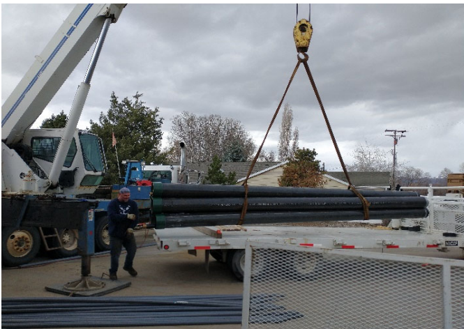
Installing new column pipe in well
