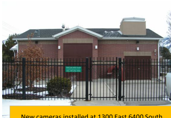
New cameras installed at 1300 East 6400 South
