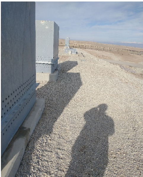
New gravel on top of new piping
