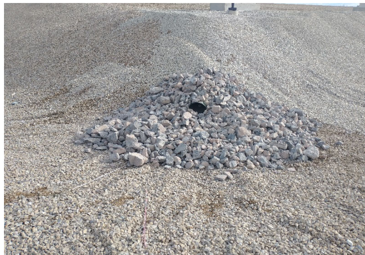
Drainage pipe at bottom corner with new riprap
