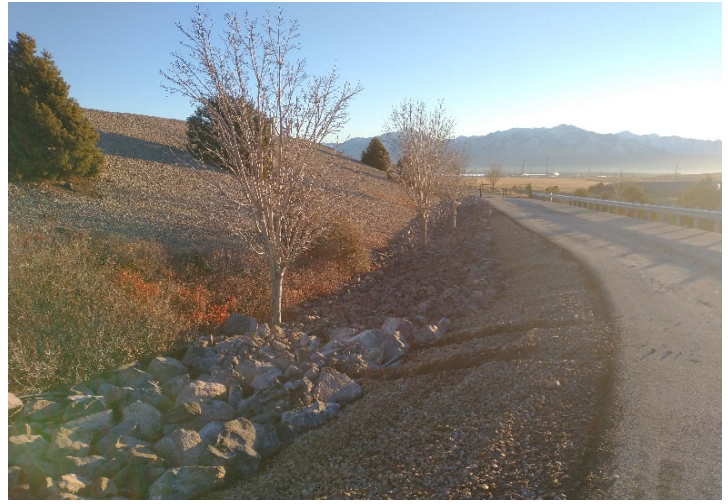
Riprap placed in channel around reservoir
