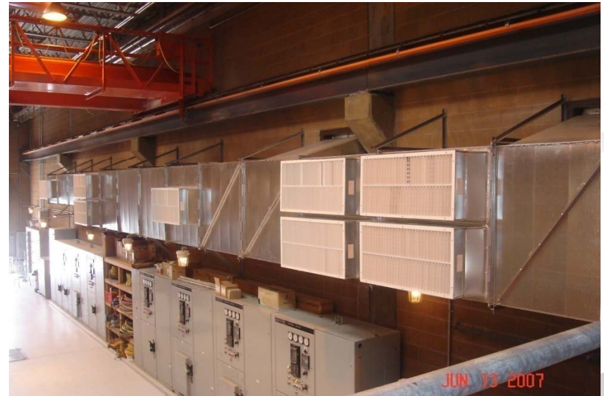
After New air distribution ducting and supply grills
