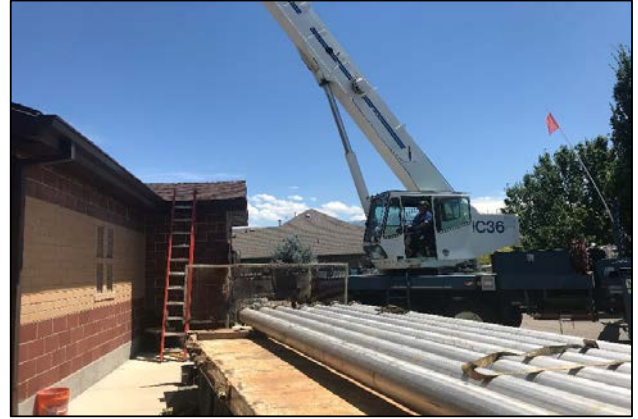
New stainless steel column pipe at DW6
