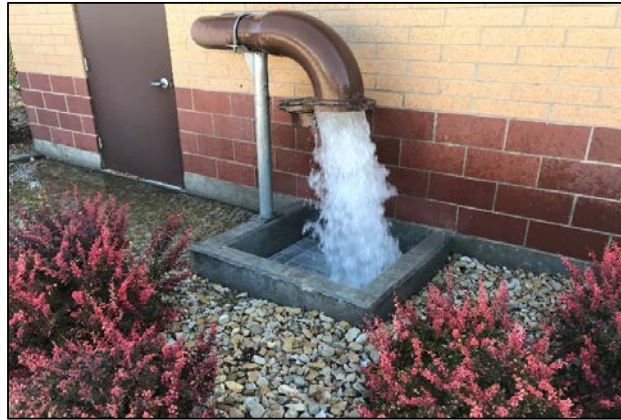
New pump testing DW7
