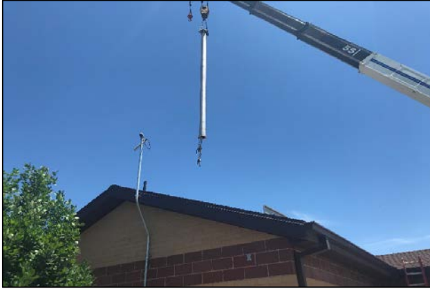
New stainless steel pump installation at DW6
