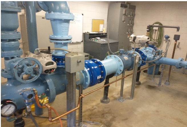
Orifice plate installed in pump-to-waste line
