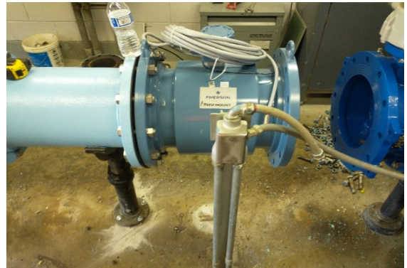
Installation of a new flow meter
