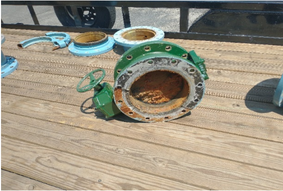
Old gate valve and other components removed from well house
