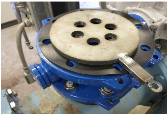
Orifice plate installed in pump-to-waste line
