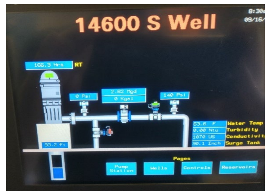
New SCADA HMI user interface screen
