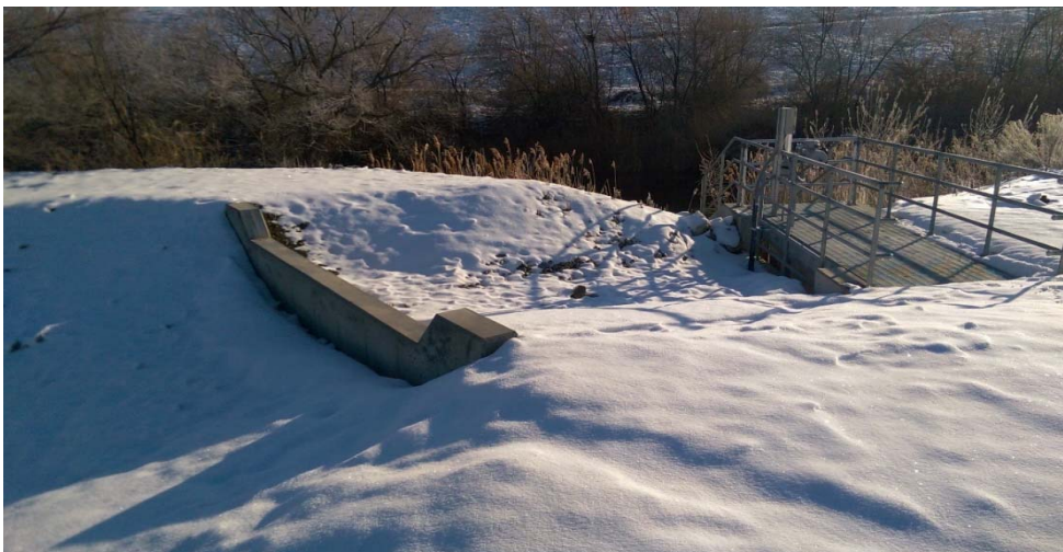
Finished Project including New Storm Detention Pond Overflow Weir
