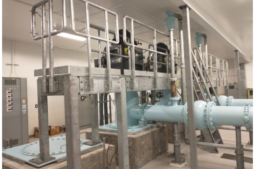
New motor access platforms
