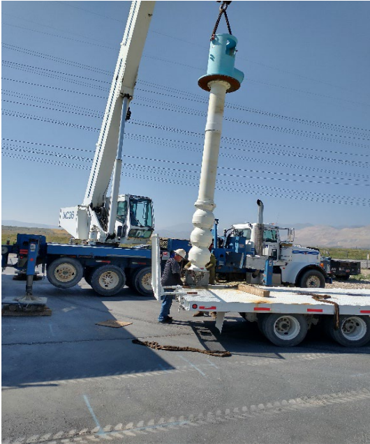
Installation of new pump
