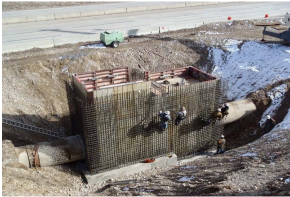
Construction of the JA-3 Chlorine Injection Vault
