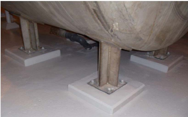
Before & After: Sleeve Valve Grout Pads
