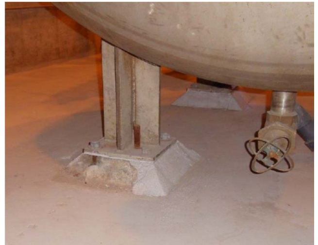
Before & After: Sleeve Valve Grout Pads
