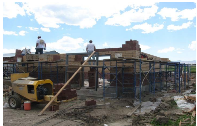
Constructing DW7 walls
