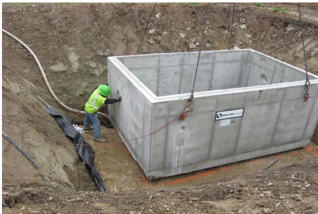
Setting DW2 precast vault
