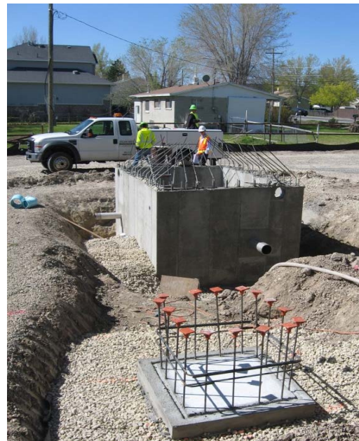
Constructing DW1 cast-in-place vault
