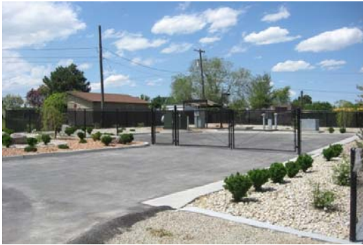
DW2 completed site
