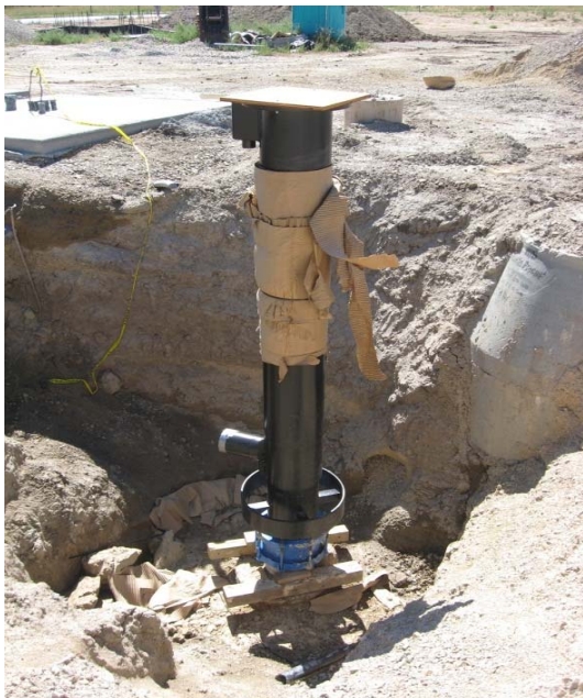
Installing DW2 pitless adapter
