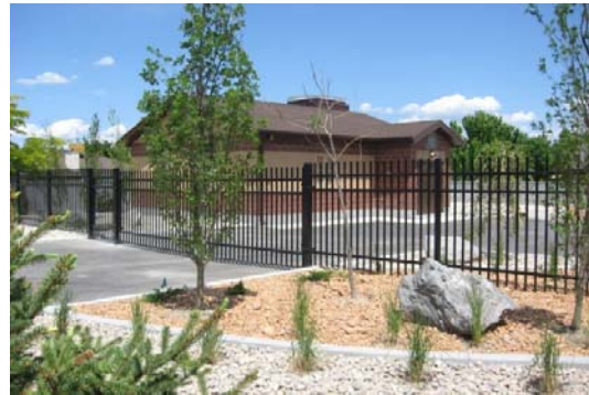
DW6 completed site
