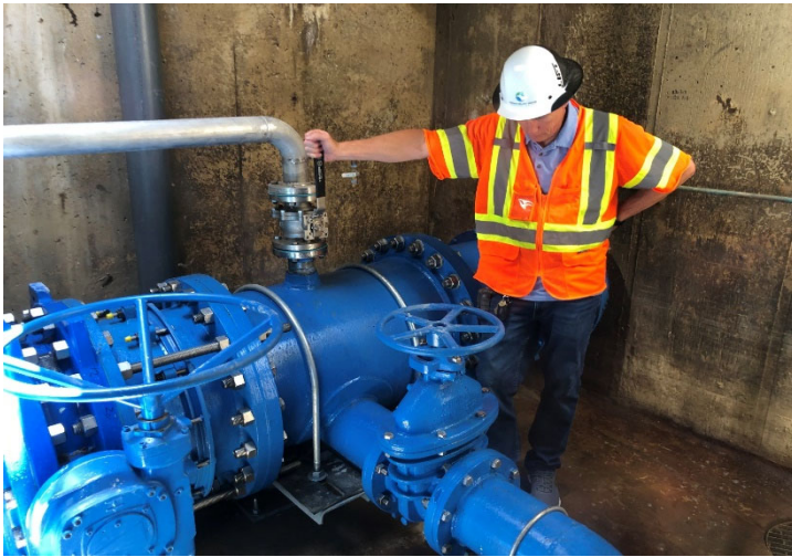
New valves and piping installed at 1175 West 4500 South mainline valve vault
