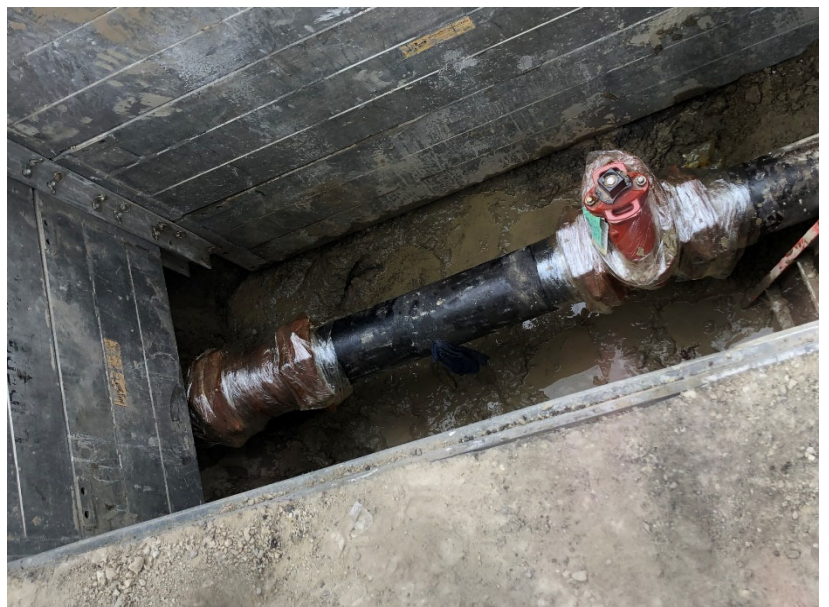
New isolation valve installed at the Gordon Lane PRV
