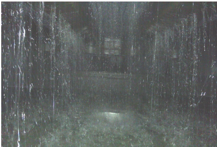
Water flow in improved air tower, showing good distribution of flow
