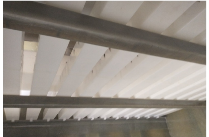
New troughs to evenly divide water flow in the air tower
