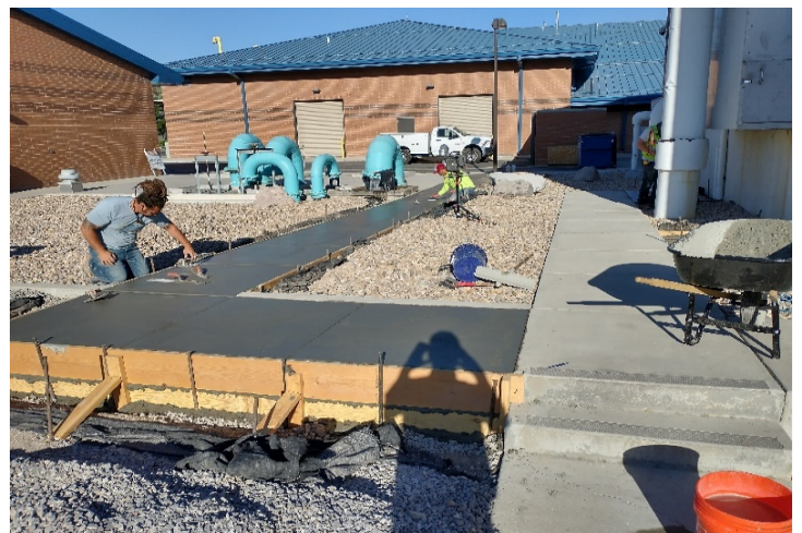
New sidewalk installed outside air tower building
