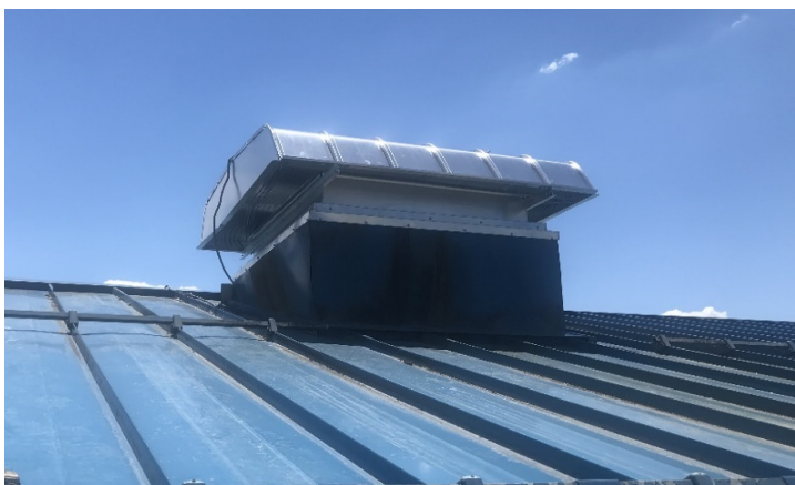
New hood installed on top of air tower
