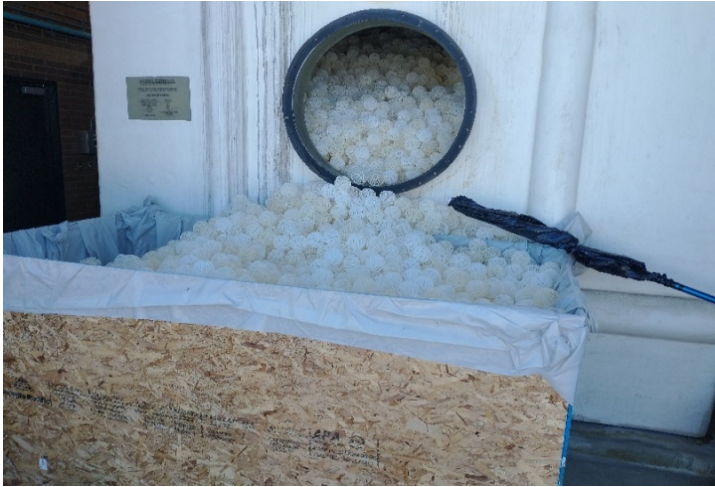
Tri-pack media balls being removed from air tower for construction inside
