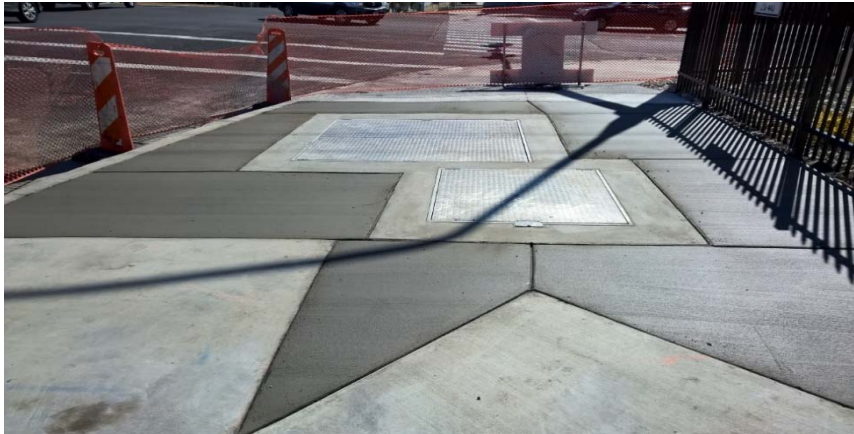
6200 South 3200 West: Vault in sidewalk
