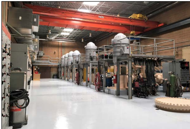
Jordan Narrows Pump Station new access hatches and newly sealed floor
