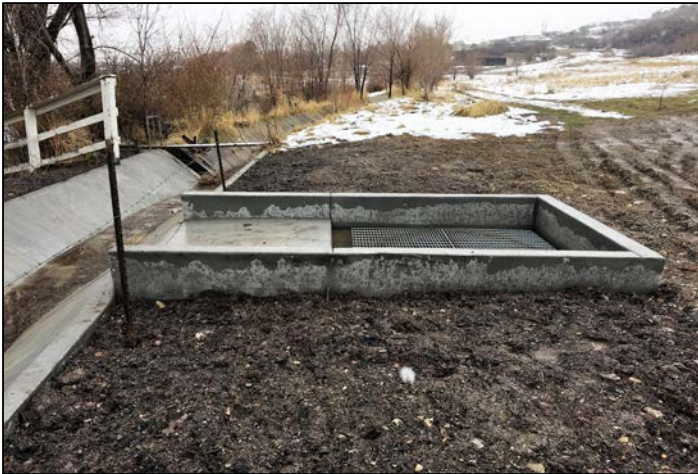
Pleasant Grove blowoff & ditch lining
