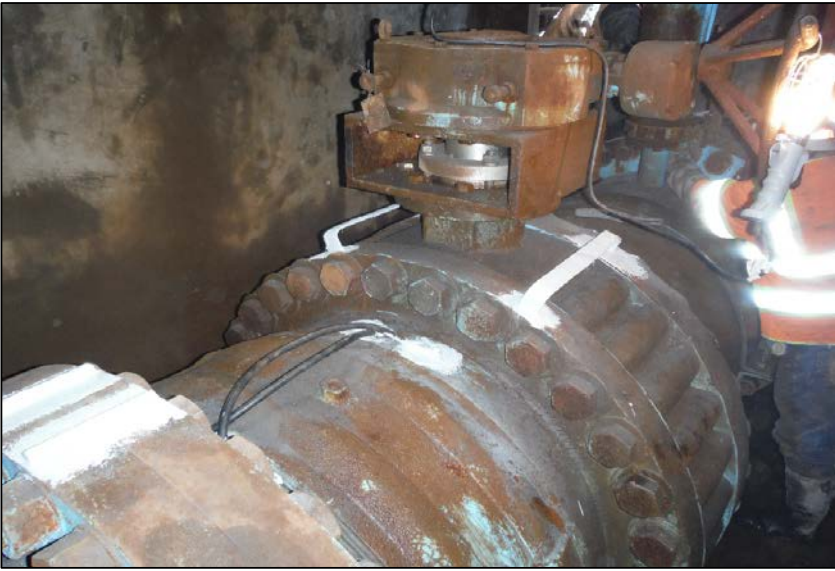
Exterior joint bond in 11400 South vault
