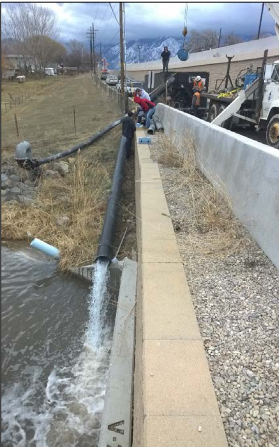
11400 South Pipeline dewatering
