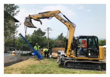
Installing line stop valve
