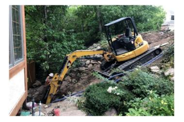
Potholing to identify location of the pipeline leak
