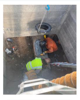
Installing welded flanged outlet
