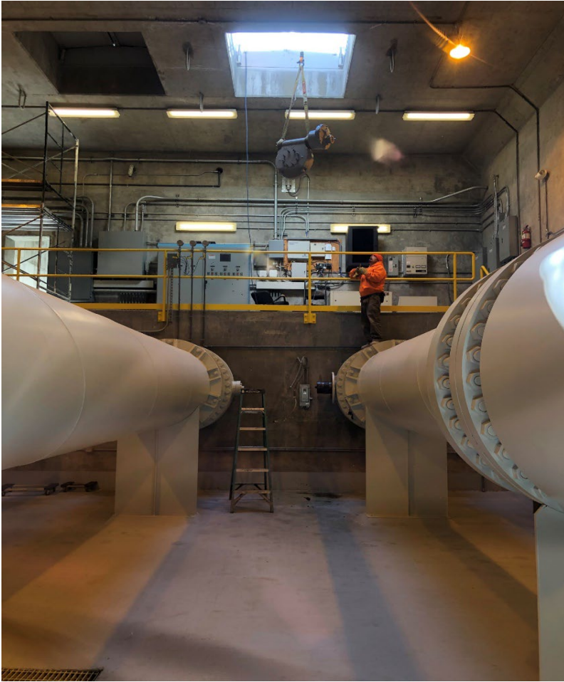
Lowering the new actuator into place at JA-4 flow control structure.
