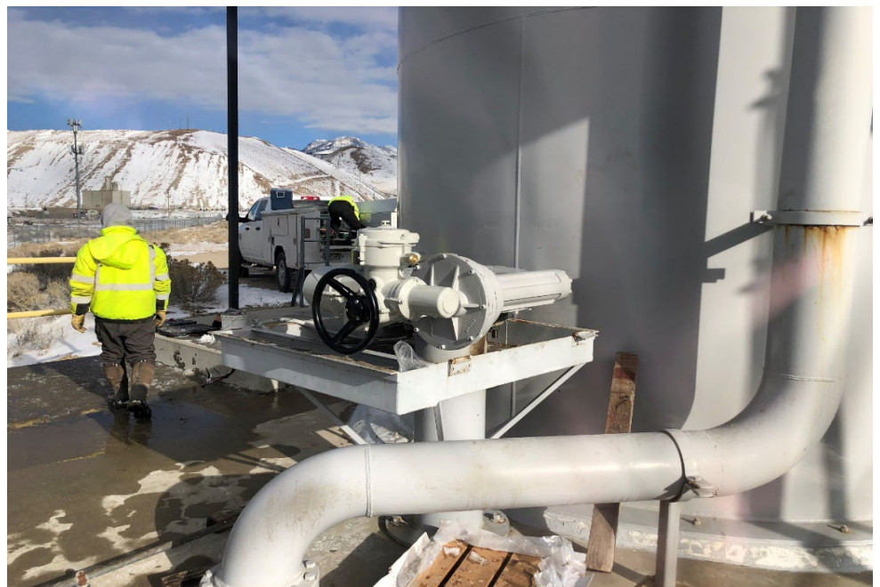
New actuator at the JA-1 standpipe.
