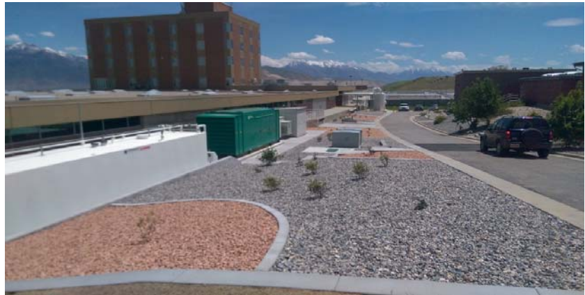
Finished project looking east
