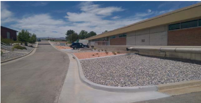
Finished project looking west
