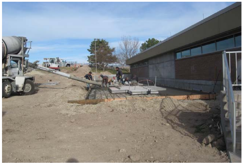
Placement of generator slab
