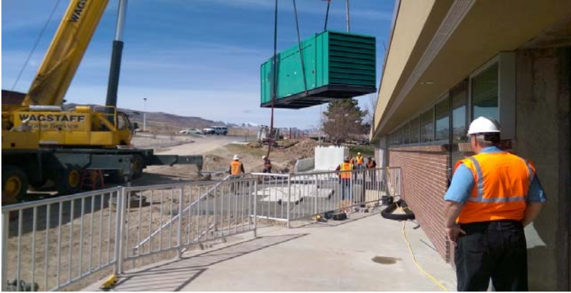
Placement of new self-contained 1000 kw generator
