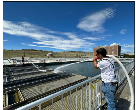
District operators washing down the plate packs
