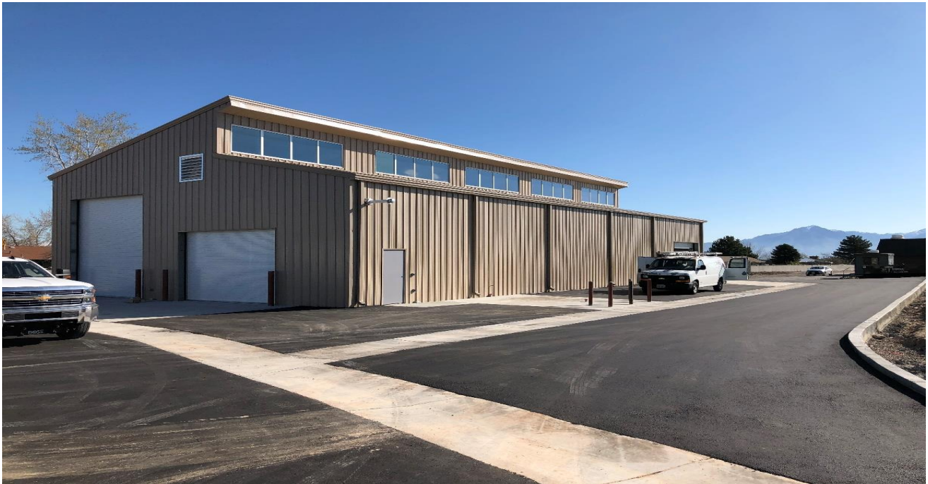
Southwest of Completed Building
