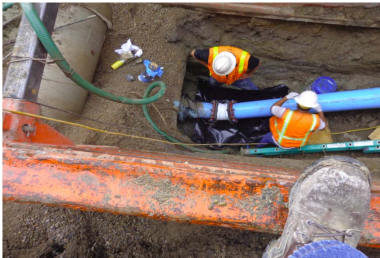
500 East Pipeline Installation
