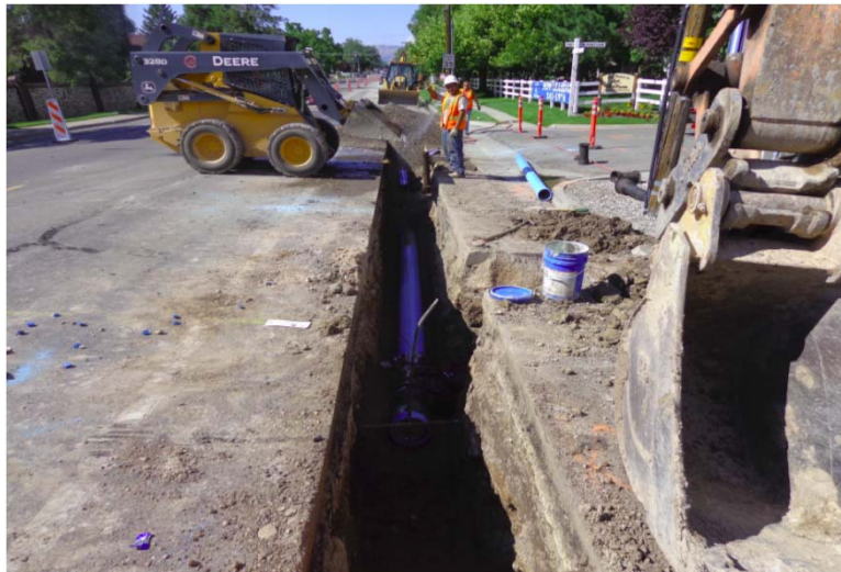
Pipeline installation at 500 East and Fox Point
