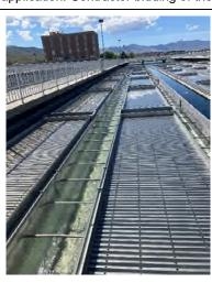
Plate settlers in operation at JVWTP
