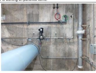
Circulation pump in vault operating new chemical feed line
