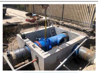
Installation of the new 30-inch piping and valves
