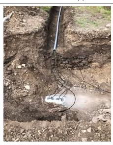
Cables cad welded to the 42-inch pipeline
