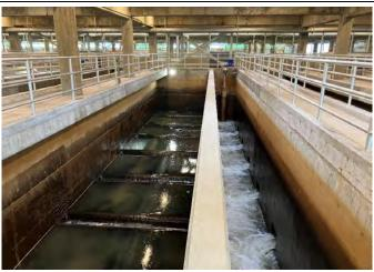
JVWTP Filter to be upgraded with deeper media and increased flow rate as part of this project
