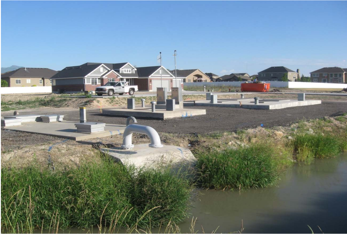
11400 South 3200 West vault site before construction.
