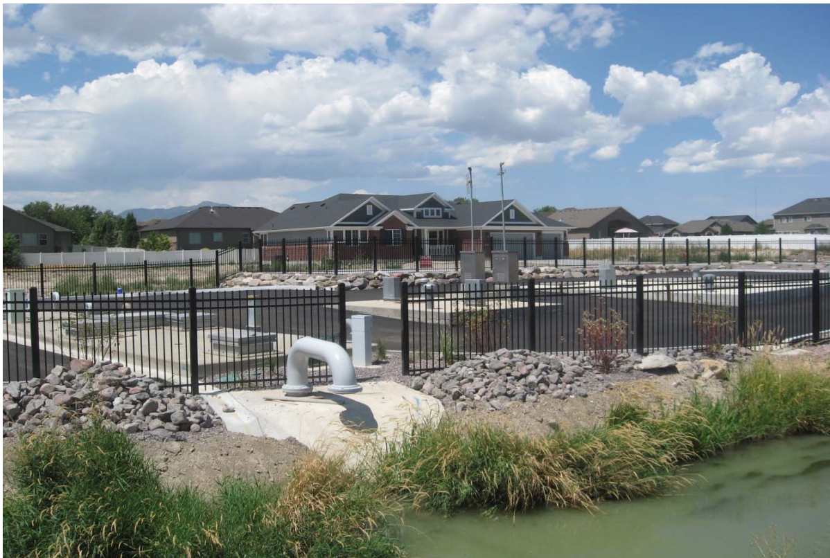
11400 South 3200 West vault site after construction.
