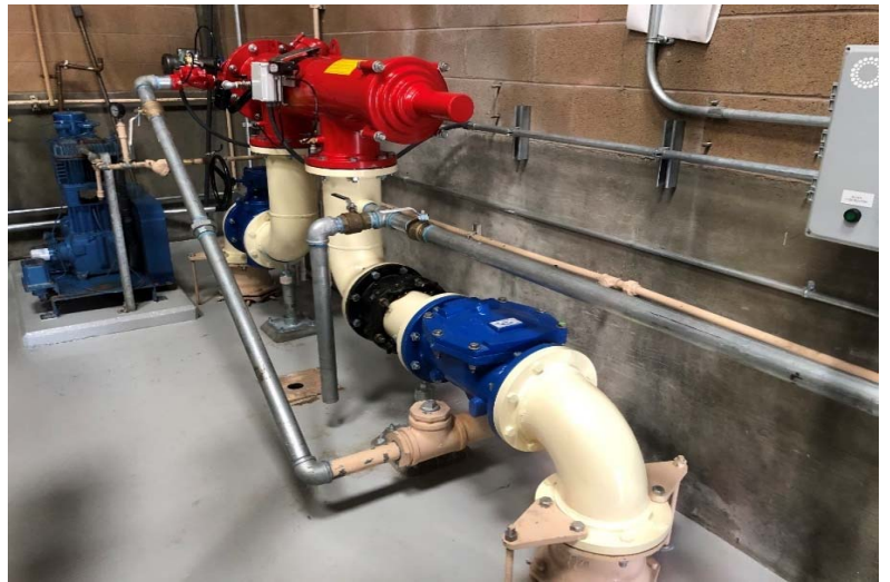
New Amiad filter for screening of process water.
