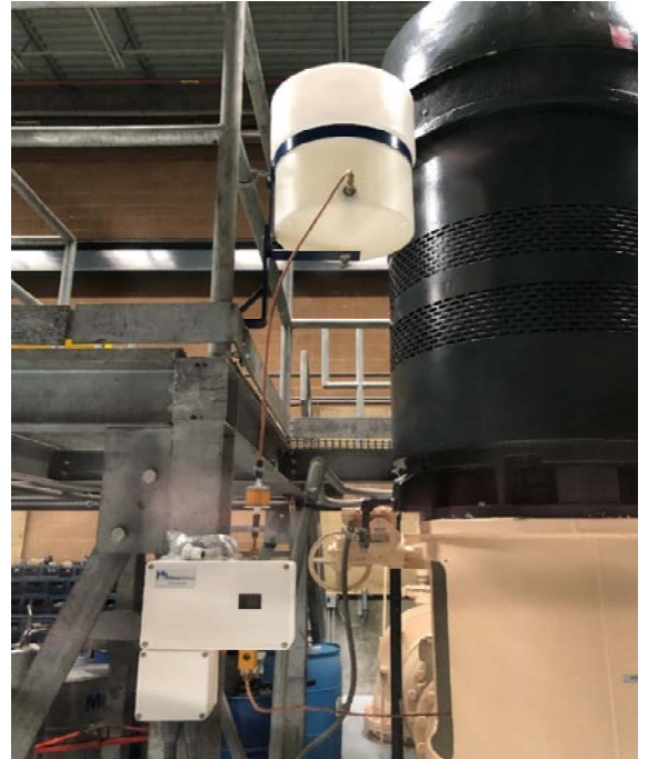
New SCADA controlled automated pump oiler.
