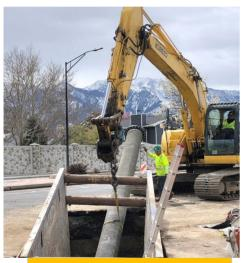
Installation of 16-inch piping at 7940 S 1300 E
