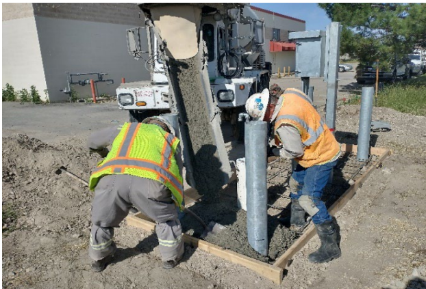
Pouring new concrete base for well, recifier, and meter pedestal
