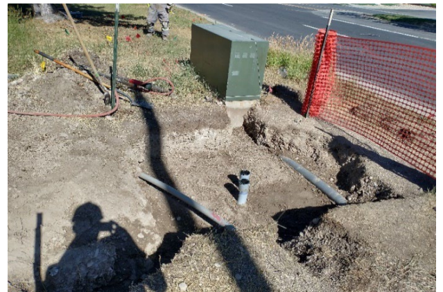
Excavated pit for new power transformer
