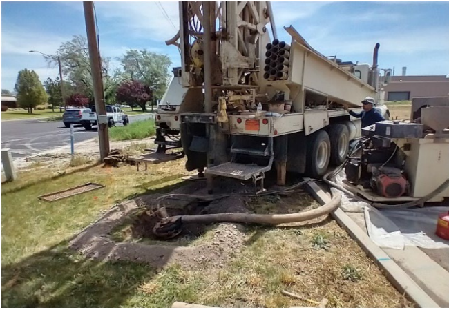
Drill rig drilling cathodic well
