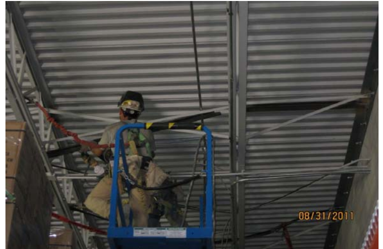
Installation of new steel angle.
