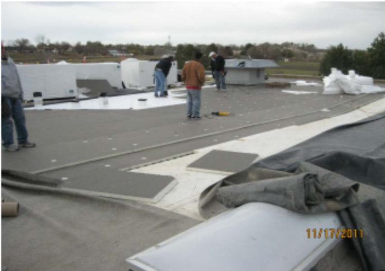
Installation of Roofing in the VSB.
