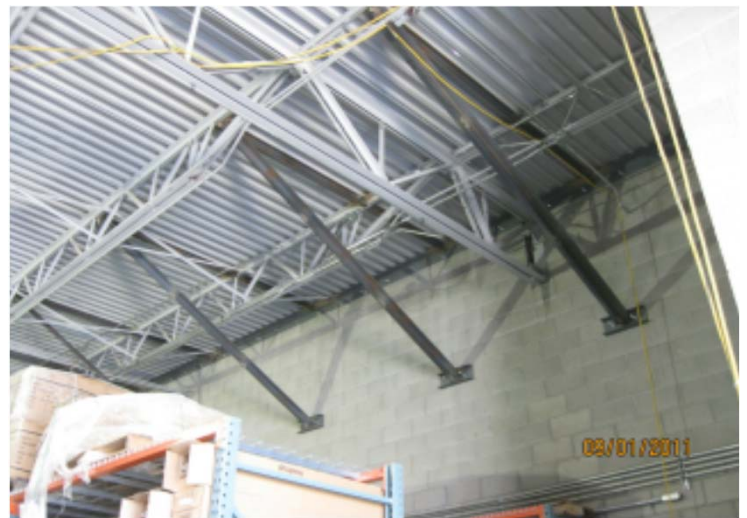
Steel kicker angle bracing installation.
