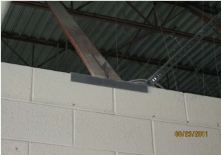
Installation of new CMU wall bracing.
