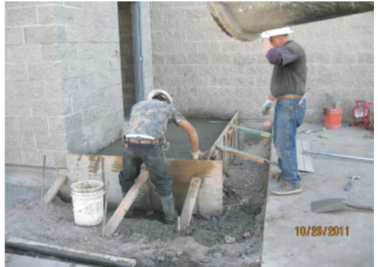
Installation of Concrete Slab at VMB Stairs.
