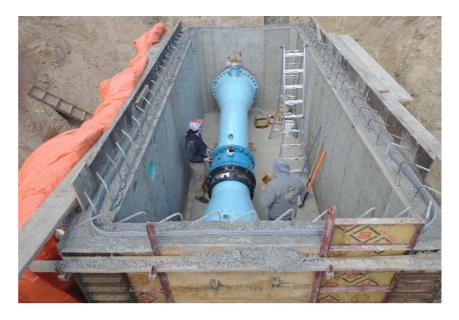
New effluent meter and piping installed in new vault
