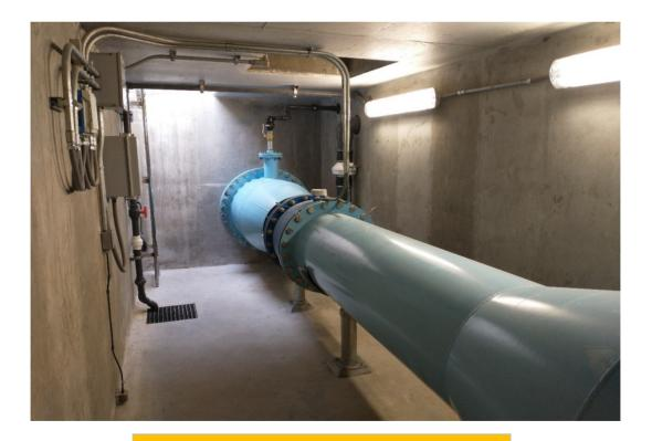
The completed meter vault with new meter, piping, ventilation, electrical, and hatches
