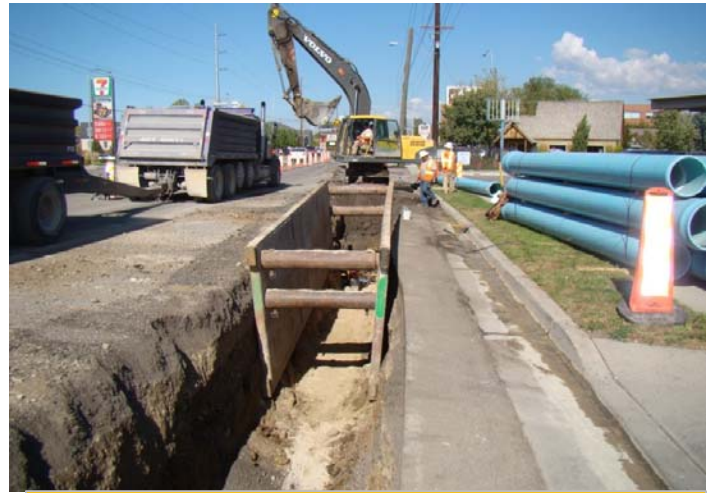
Open trench installation
