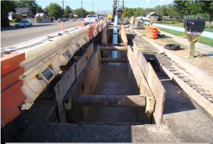
Directional drilling near Wheeler Farm
