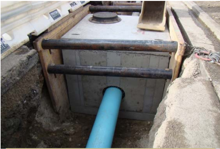
Placement of a new valve vault
