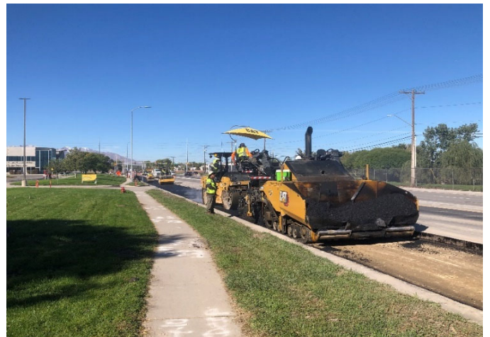
Asphalt placement
