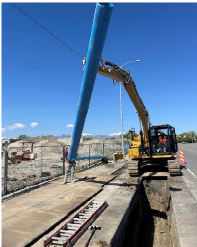
Installing new 12-inch pipeline
