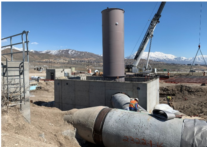
POTM new standpipe during construction
