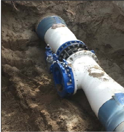
Connection to Existing Pipeline
