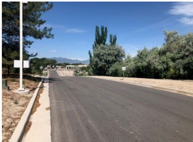
Beckstead Lane roadway improvements
