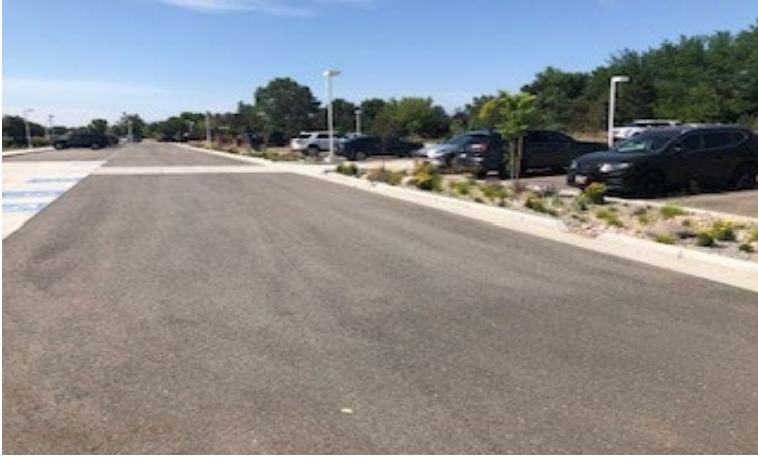
West parking area of Admin Building
