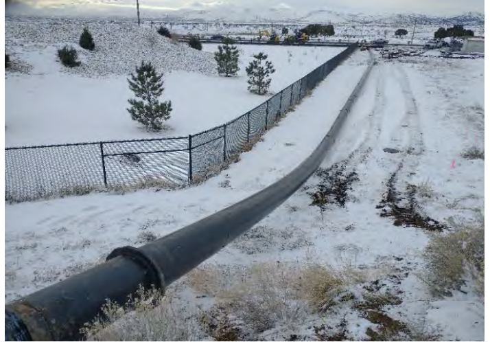
Laying new HDPE line
