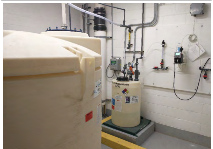
Chlorine Feed System in New Chemical Building
