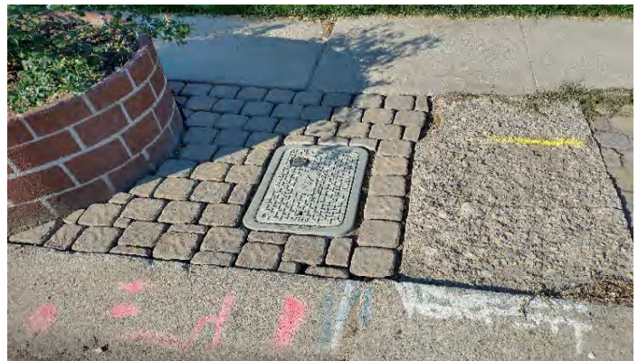
Completed new service connection box
