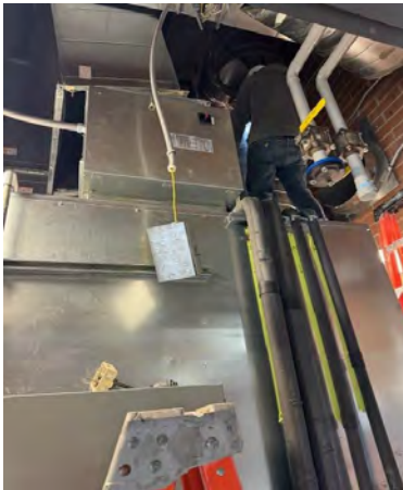
RO Plant Duct and Pipes Installation
