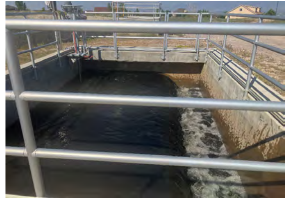
JWTP Backwash waste water during feeding of activated carbon powder
