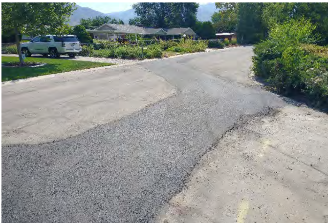
New asphalt over new pipeline
