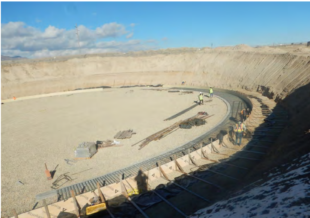
Setting forms and rebar for the East Tank footings
