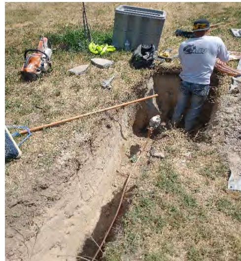
New setter installed in yard
