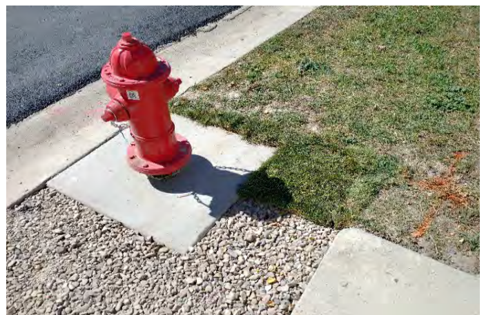
New hydrant with concrete pad and new landscaping
