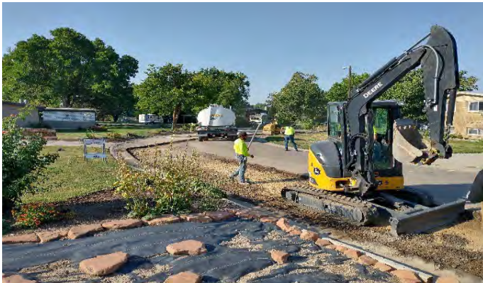
Compacting on top of new waterline
