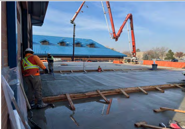
Access to Bldg Concrete Driveway
