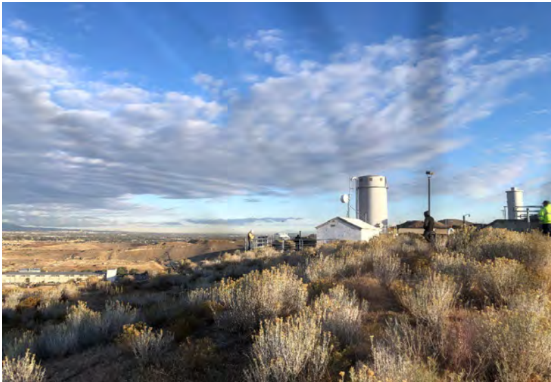
JA geologic inspection at POTM
