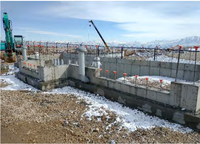
Laying walls and vents for new building
