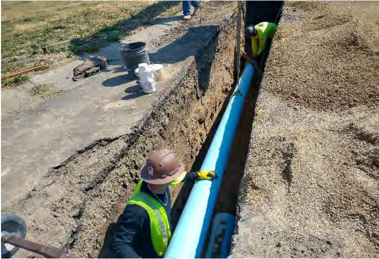
Laying new 8-inch PVC pipe
