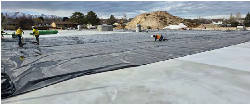
Prepping the roof deck for cover
