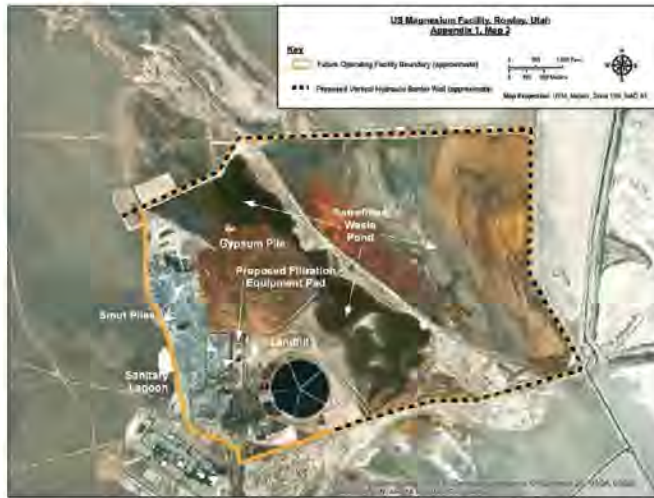
This map, filed in federal court in Utah in 2021, shows the approximate outline of a retaining wall required at US Magnesium under the company's settlement with the Environmental Protection Agency.
