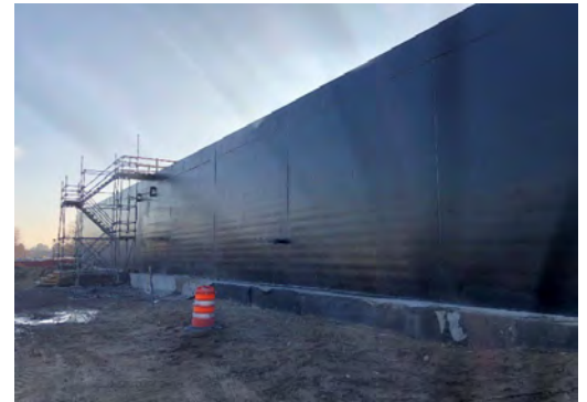
Waterproofing applied to the reservoir wall
