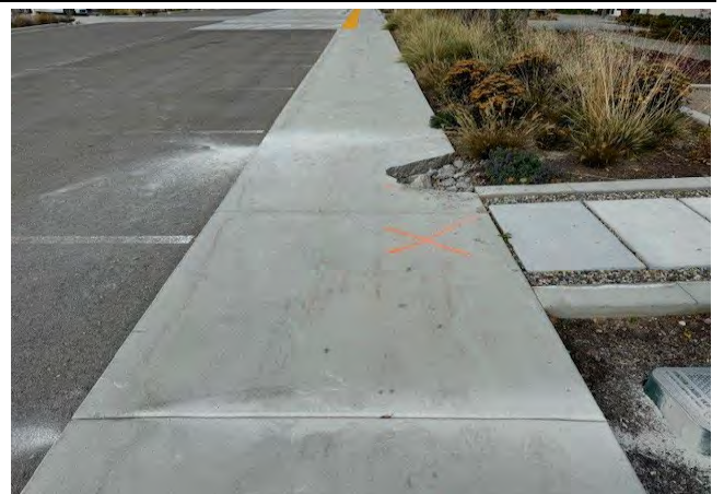
Sidewalk Prep Concrete Replace
