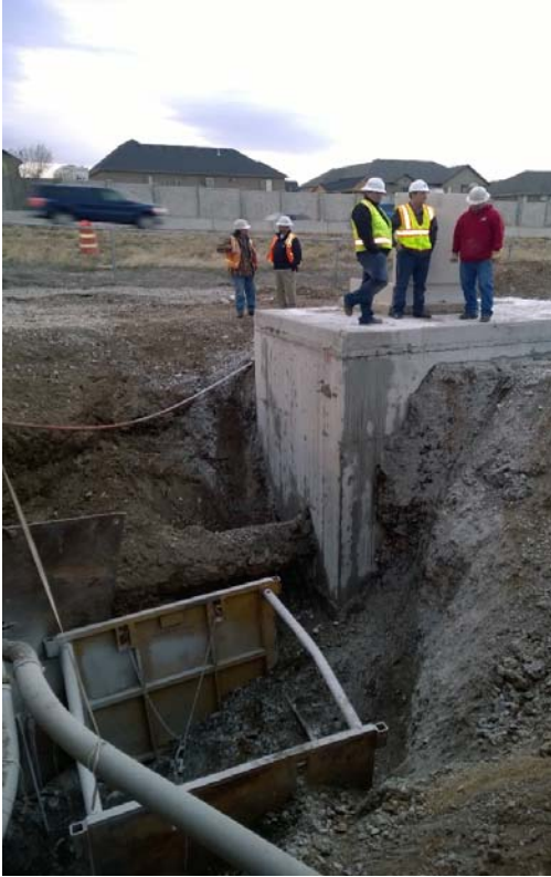
Excavation for new meter vault
