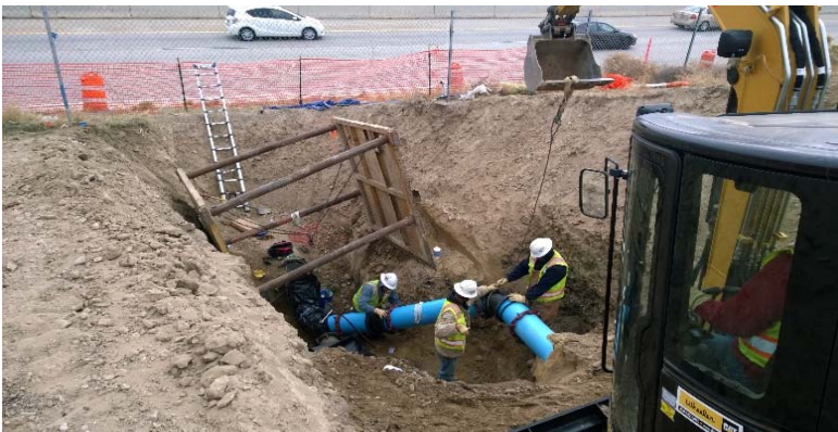
Excavation for new meter vault
