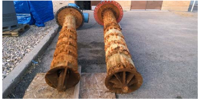
Old pumps removed
