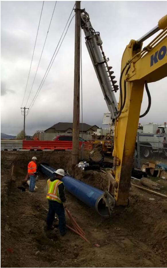
Pipe installation under Bangerter Highway
