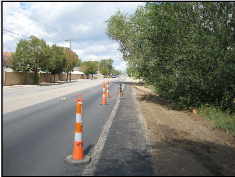
Finished construction on 1300 West.
