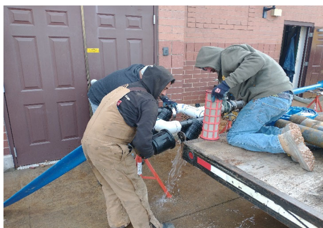
Filtering well water to look for gravel
