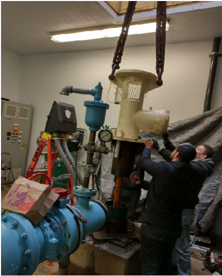
Pulling the pump and well head
