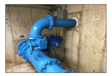
Recoated Piping in the Utility Meter Vault
