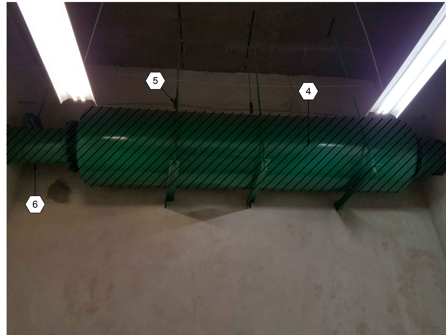
DISCHARGE SILENCER PHOTO B 3M-101
