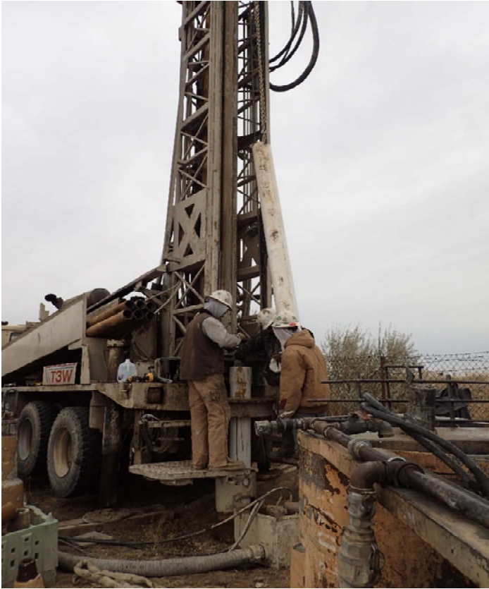
Drilling anode well
