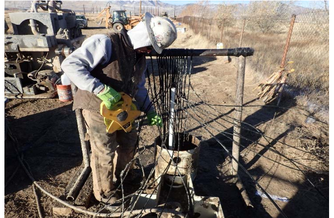
Setting anodes in anode well
