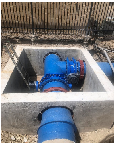
New piping installed within vault
