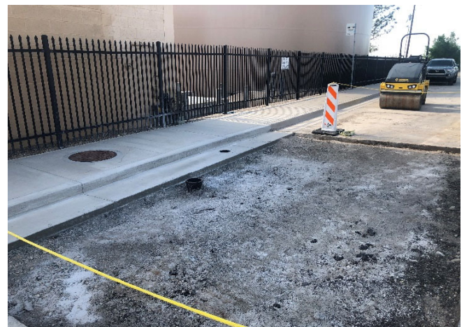
Preparing for asphalt placement
