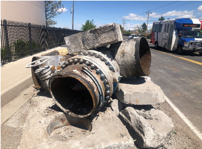
Demolition of vault lid, piping, & valves
