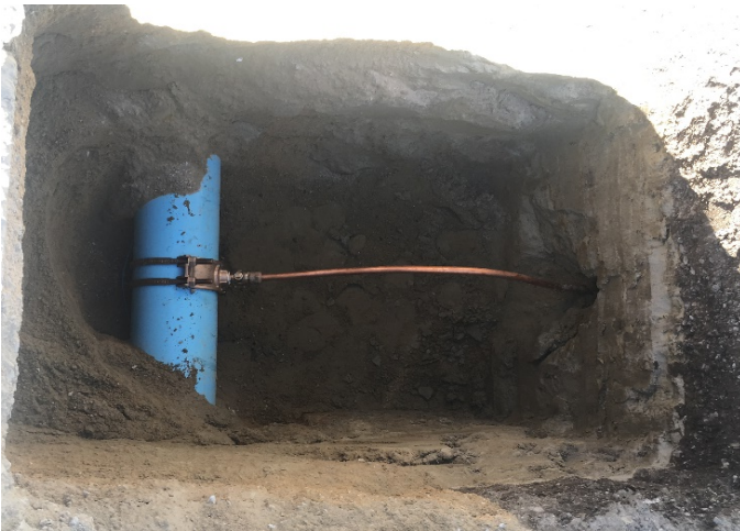
New 3/4" service connection.
