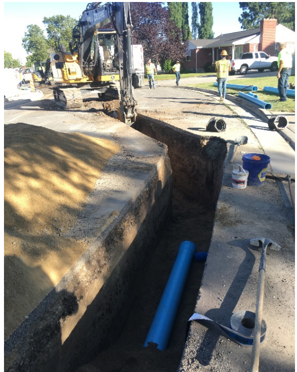
Installation of the 8" pipeline along Julep Drive.
