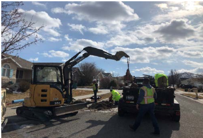
Replacing valves in the Foothills subdivision.
