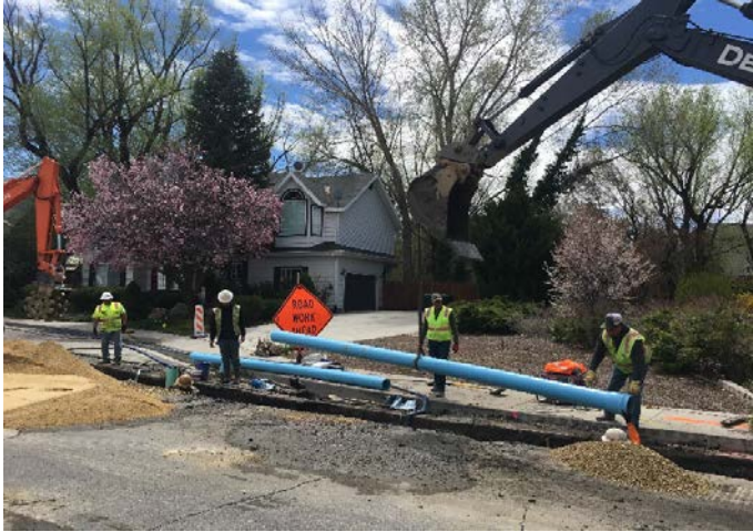
Installation of the 8" pipeline along Creekview Drive.
