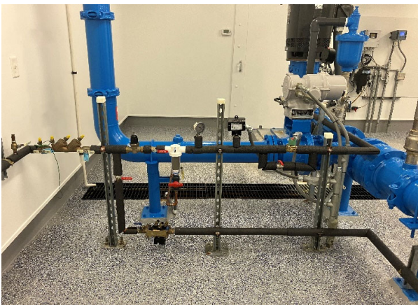
New water "pre-lube" piping (flushes well with city water prior to start up to wet the marine bearings) and reconditioned discharge head/motor awaiting start-up
