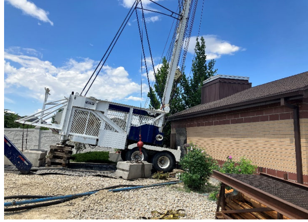
Well Redevelopment Machine
