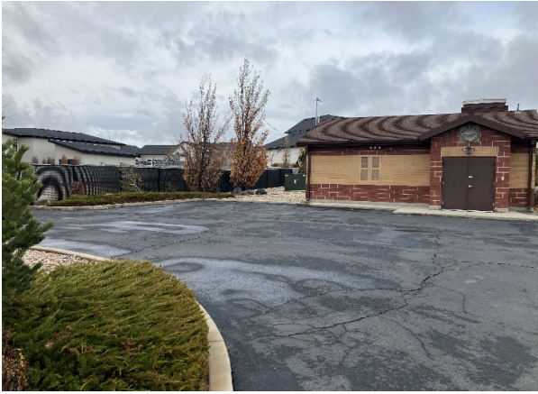
DW7 Well Pump House
