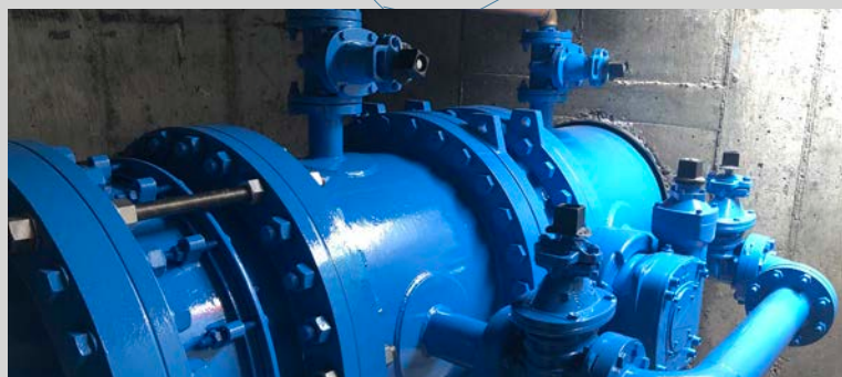
Refurbished vault at 2200 W and 6200 S
