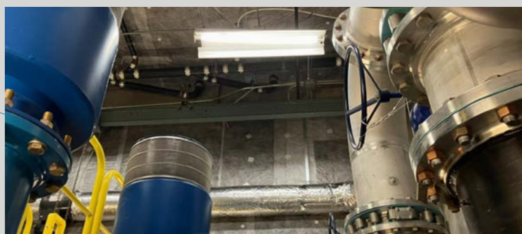
JWTP Blower Room Acoustical Improvements
