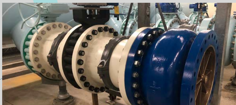
11800 South Pump Station Upgrades
