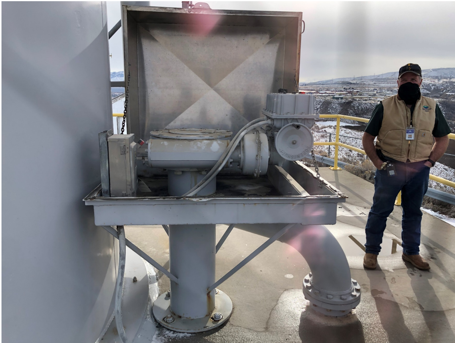
Figure 10: Existing 78-Inch Butterfly Valve Actuator
