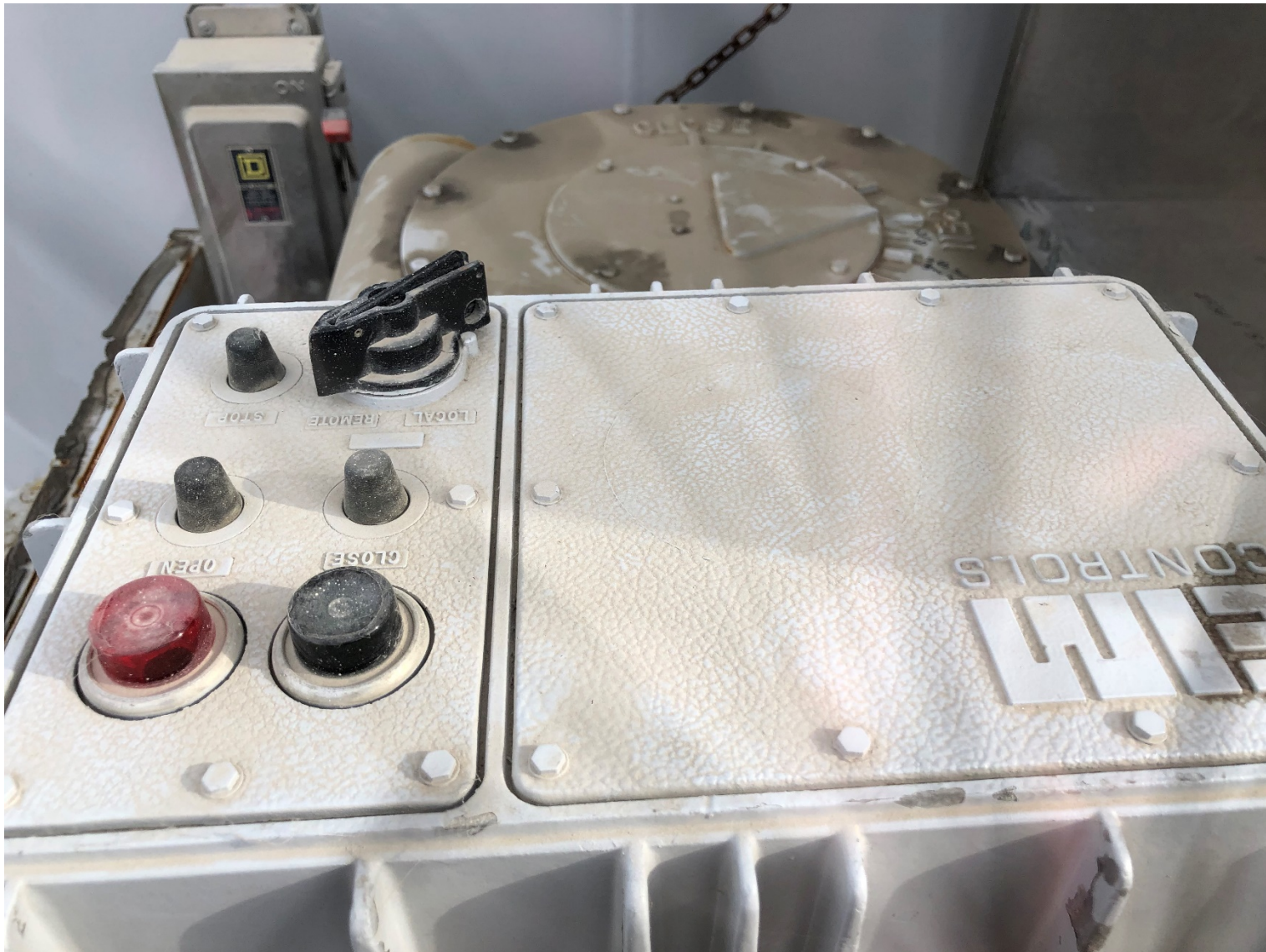
Figure 11: Existing 78-Inch Butterfly Valve Actuator Controls (Inside Enclosure)
