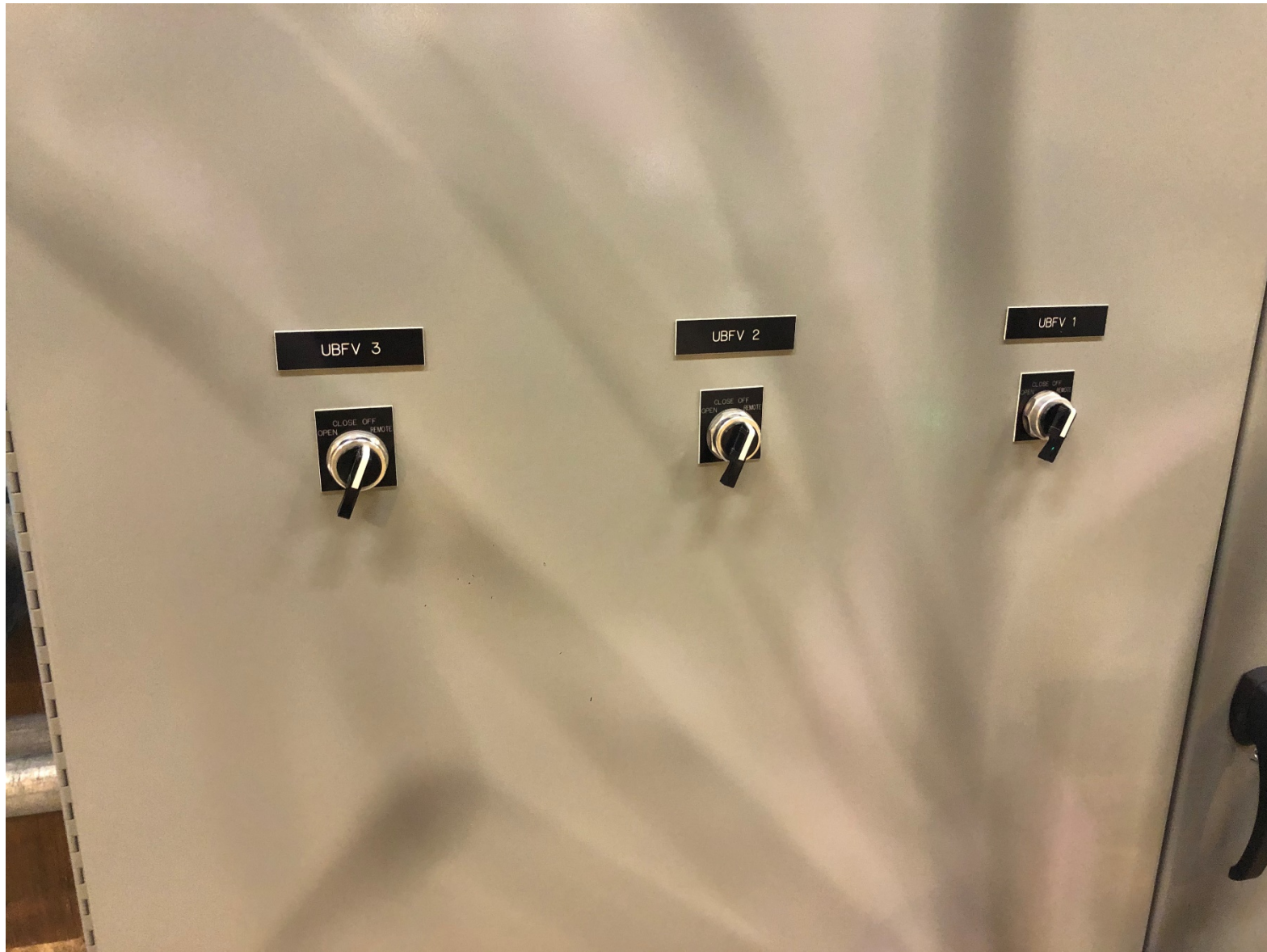
Figure 2: 42-Inch Butterfly Valve Hand Controls on Upper Mezzanine
