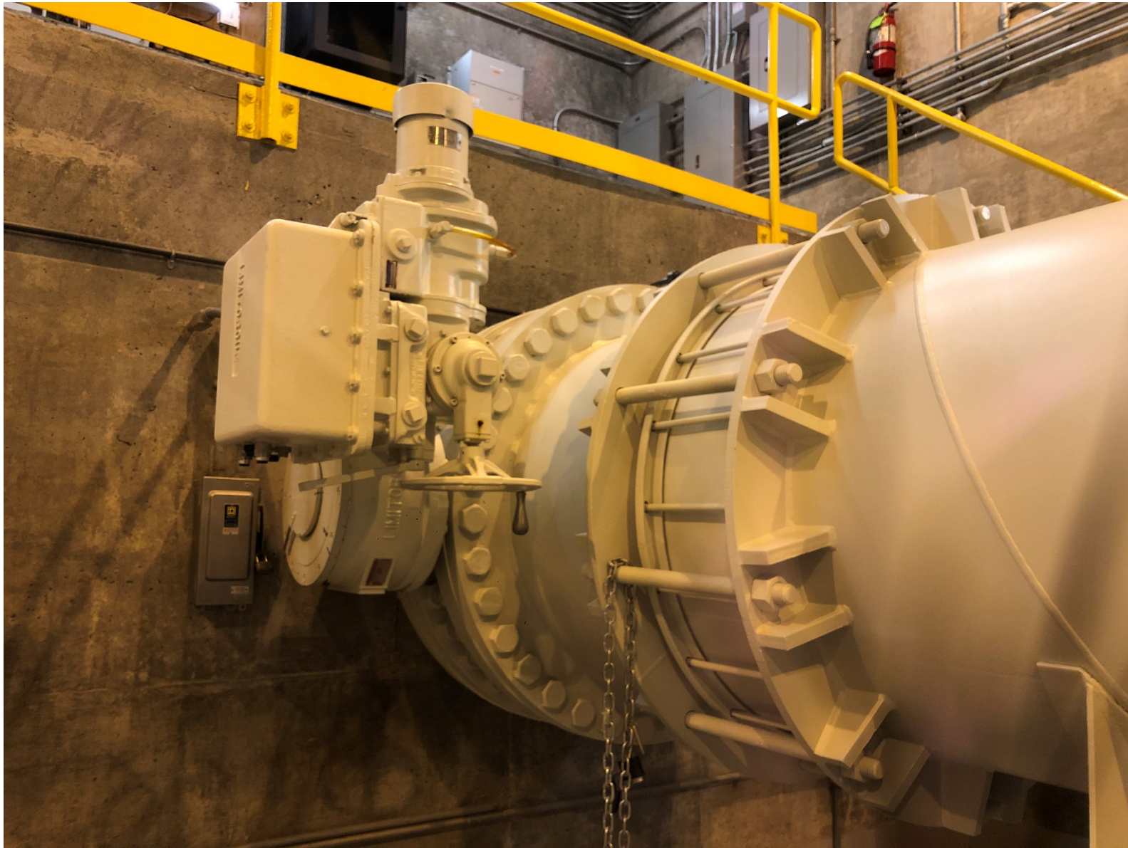
Figure 1: Existing Actuator and Gear Box on 42-Inch Butterfly Valve
