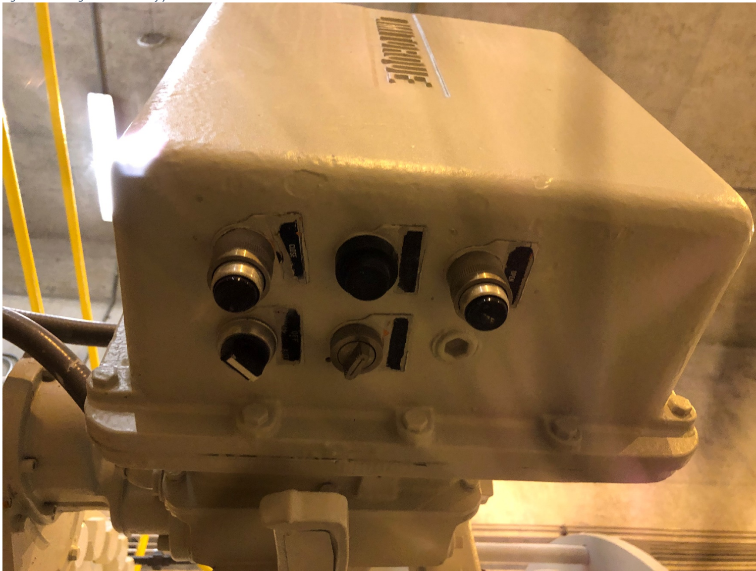
Figure 5: Existing 42-Inch Butterfly Valve Actuator Controls
