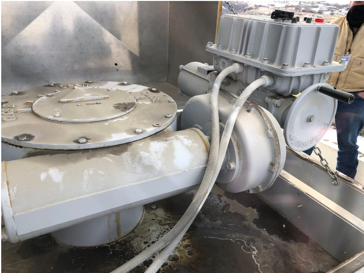
Figure 12: 78-Inch Butterfly Valve Actuator
