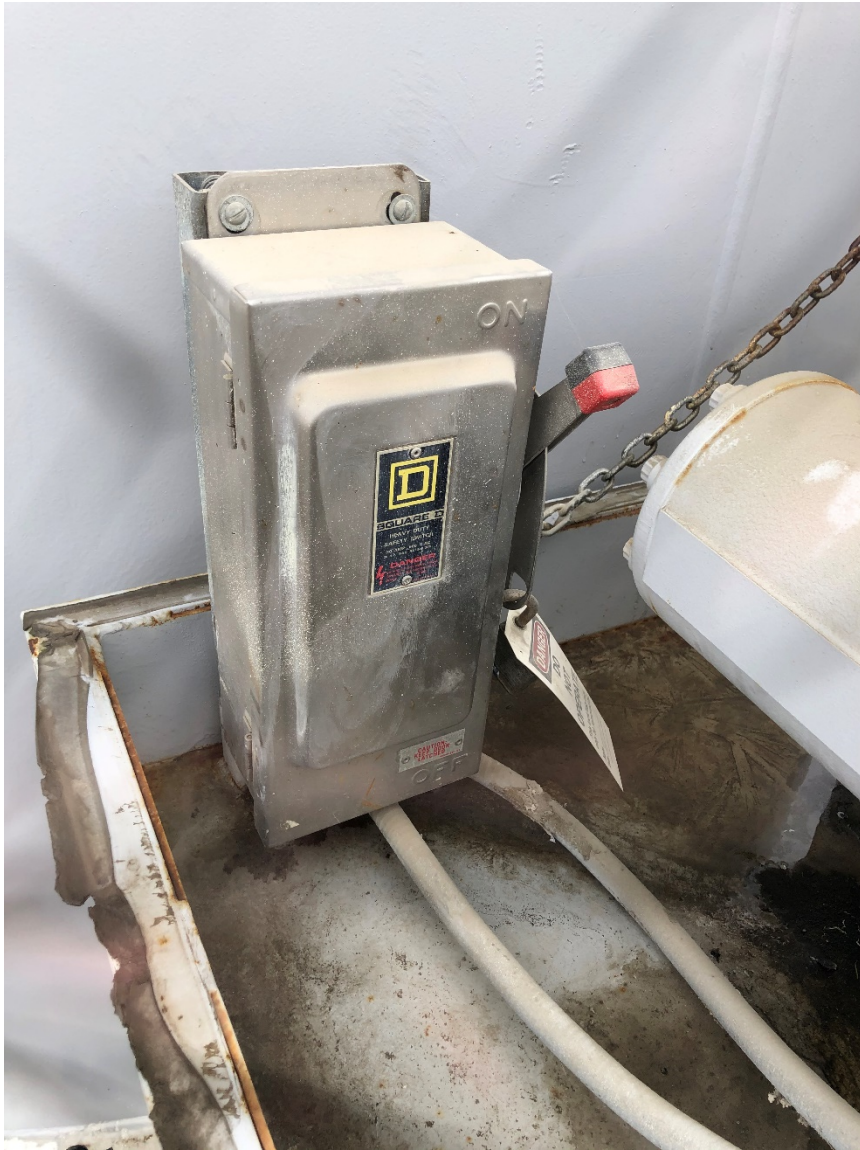
Figure 13: 78-Inch Butterfly Valve Actuator Electrical Disconnect
