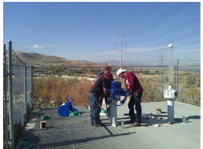
Installing New Actuators
