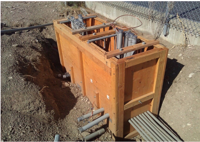
RTU Base Frame Ready For Concrete
