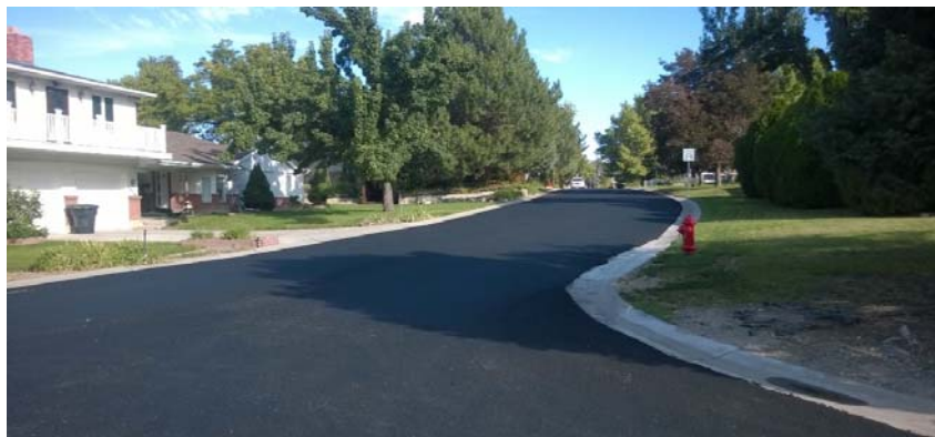
935 East Slurry Seal Asphalt Coating
