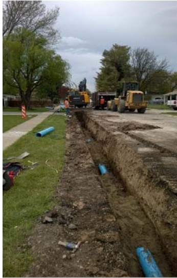
Pipe Laying Along 5190 South
