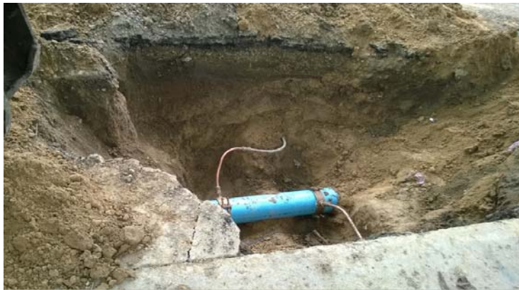
5235 South Service Reconnections
